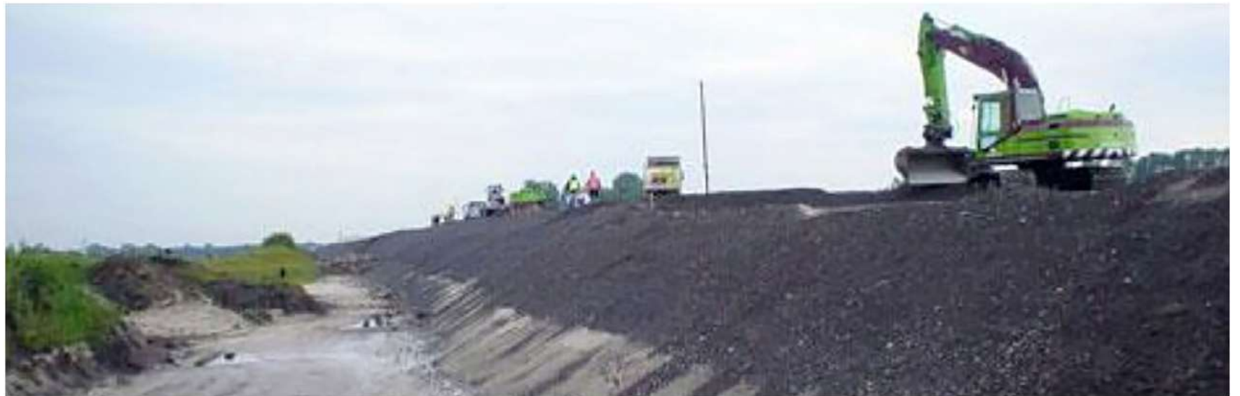
Figure 24 Construction of noise barrier along the A12 highway in The Netherlands.
