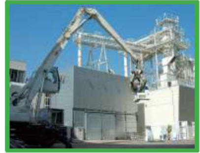
▲ Heavy equipment operations before shredding
