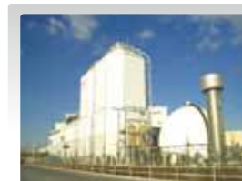
Facility for biogas power generation
