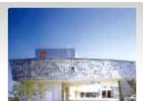
Recycling facility for E-waste
