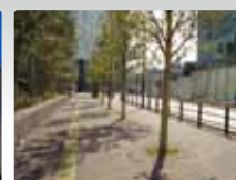
Example of Eco-cement usage (Interlocking block)
