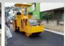
Usage of slag (asphalt pavement)
