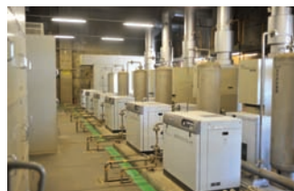
Micro-gas turbine generator
