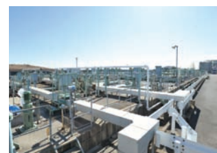
Wastewater treatment plant No.3
