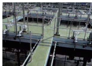
Wastewater treatment plant No.1
