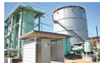
Facilities related to gas collection
