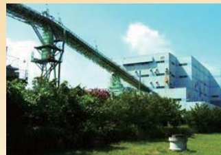
Central Breakwater treatment center for non-combustible waste
