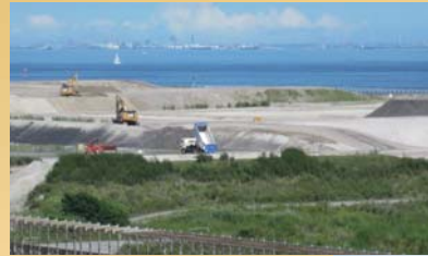
Work at the Central Breakwater New Sea Surface Disposal Site
