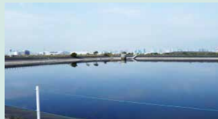
When the rain falls on the landfill site, it goes through layers of waste and flows into Buffer Reservoir which adjust the volume and quality of the water. Finally, it's sent to Wastewater Treatment Plants.
