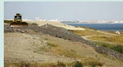
Central Breakwater Outer Landfill Site
