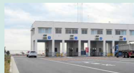
Solid waste bound for landfill is measured and registered its weight at the gate to the New Sea Surface Disposal Site.
