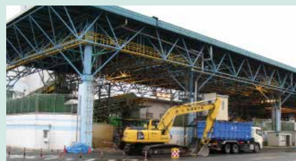
Bulky household waste is pulverized in the Pulverization Processing Plant for Large-size Waste on the Central Breakwater Inner Landfill Site.
